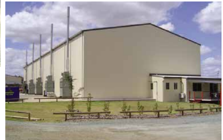
South Carolina USA Facility
