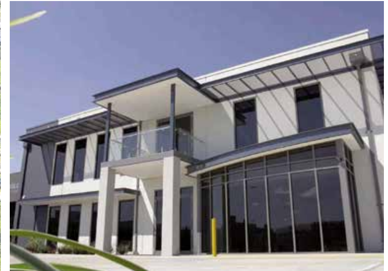
Forrestdale WA Facility
